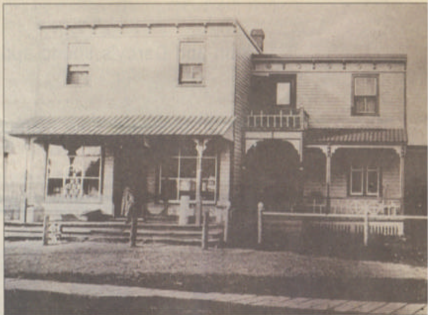
Original store burned to the ground in August 1948 when a rubbish fire got out of hand. A week later, the family was back in business.
