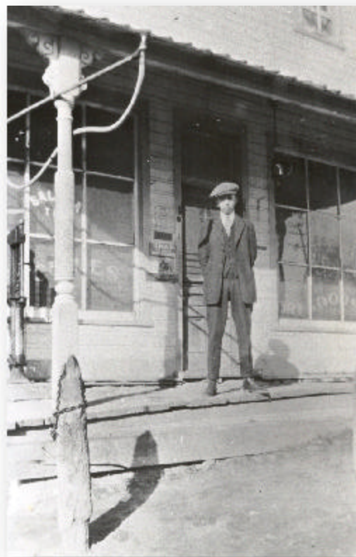
Morris Bradley in front of the old store
