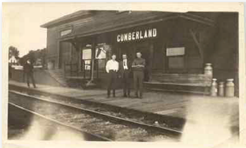
The Cumberland Station was built in 1908-9 but had a short active life. In 1915, Canadian Northern replaced the agent with a caretaker. By 1931, when passenger service on the line ended, it was a flag station only.
