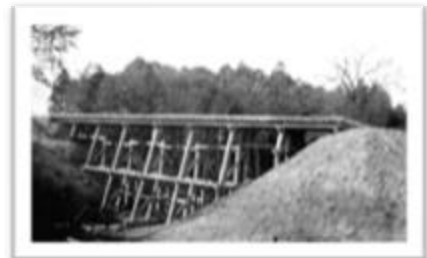
Railway bridge over Taylor Creek (contributed by Kim Taylor)
