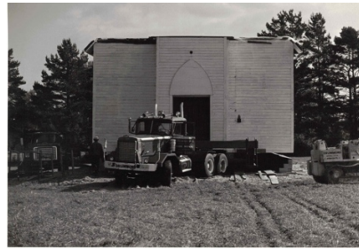
1980: The steeple and roof trusses were removed; the Sunday School and kitchen addition were removed from the rear of the building, and the main body of the church became a basic box-like structure. The steeple and roof trusses were transported separately. After placement on site at the Museum its interior plaster work was repaired.
