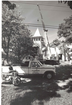
1980: The steeple and roof trusses were removed; the Sunday School and kitchen addition were removed from the rear of the building, and the main body of the church became a basic box-like structure. The steeple and roof trusses were transported separately. After placement on site at the Museum its interior plaster work was repaired.
